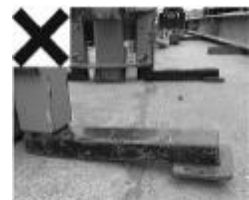
Damage to the Stability legs causing the Pipe Lifter to become unstable.
